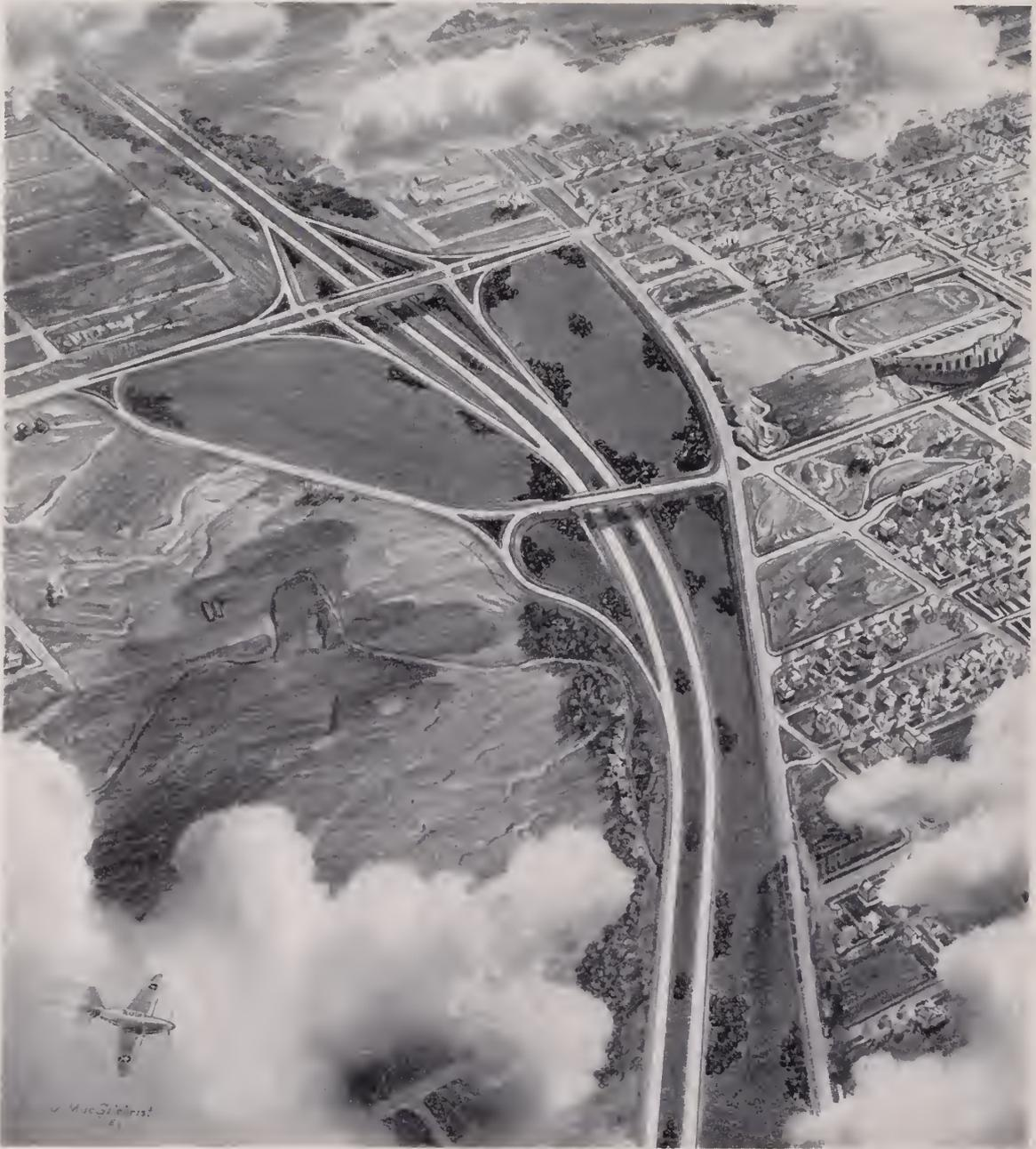
FIG. 27—At the southern terminus of the Denver Project, the Valley Highway is to have ramp connections to University Boulevard, which crosses the sketch near the top. A few blocks to the west, a bridge across the Highway would handle traffic concentrations coming from the parking area of Denver University's stadium.
